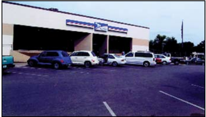
The current Milton Post Office on Dogwood Drive.
