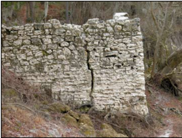
Today, the coquina walls of the springs are cracked and eroding into the Suwannee River.
