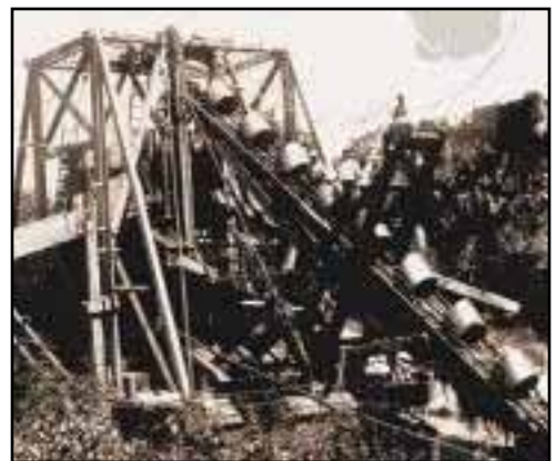
Figure 4 Early dredges were made of steel buckets attached to continuous steel chain.
